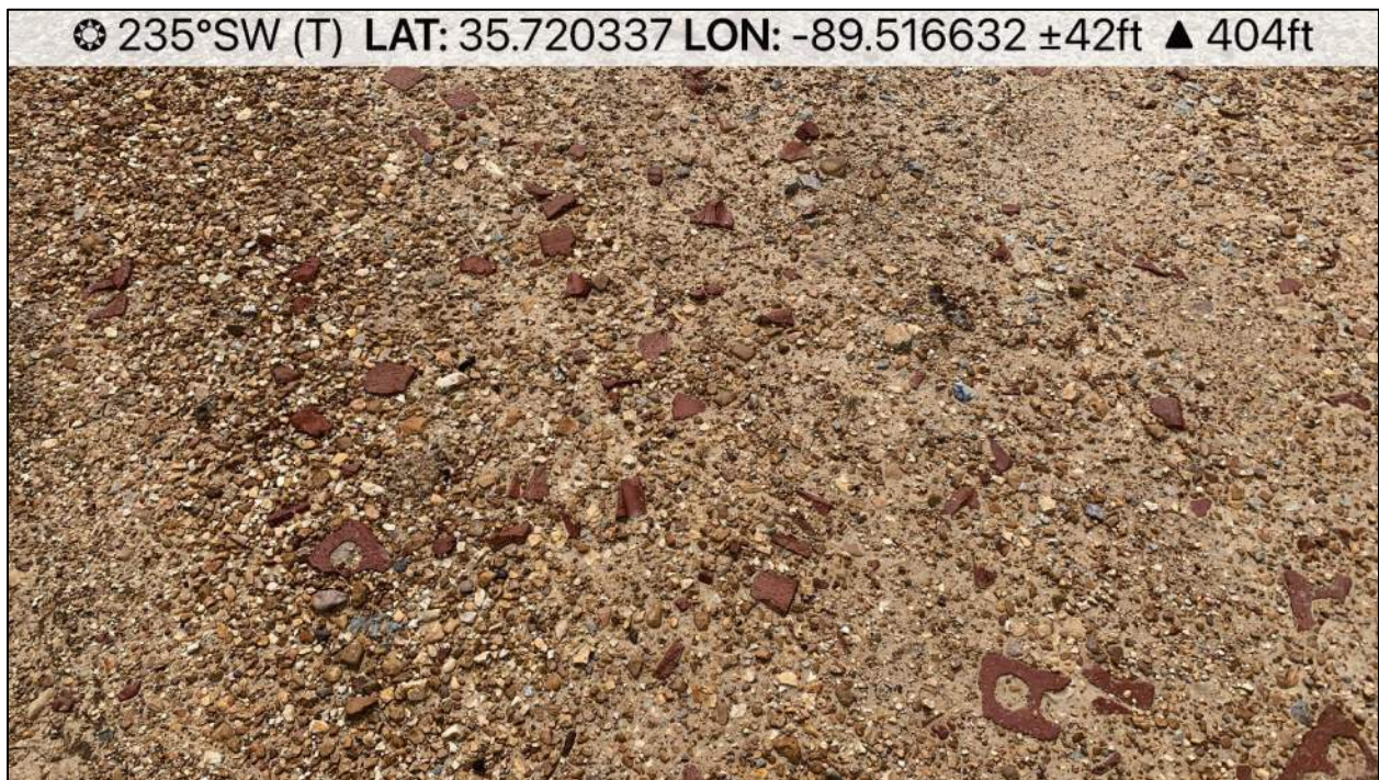
Photo 20 Brick debris in gravel along access route.
