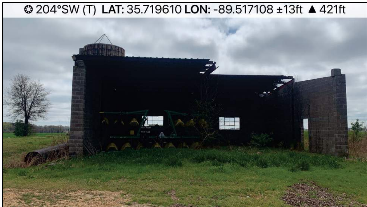
Photo 10 Facing southwest, view into farm equipment storage building.
