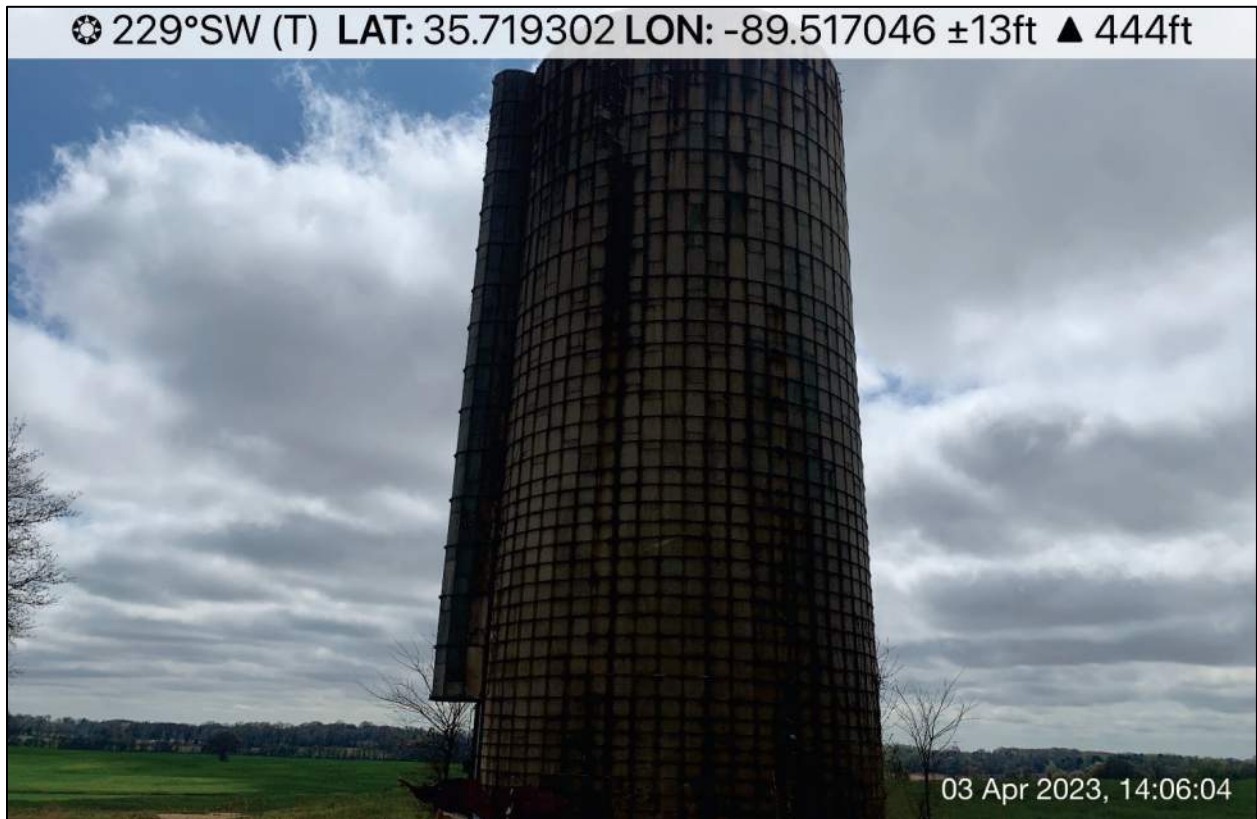
Photo 16 Facing southwest, unused silo.
