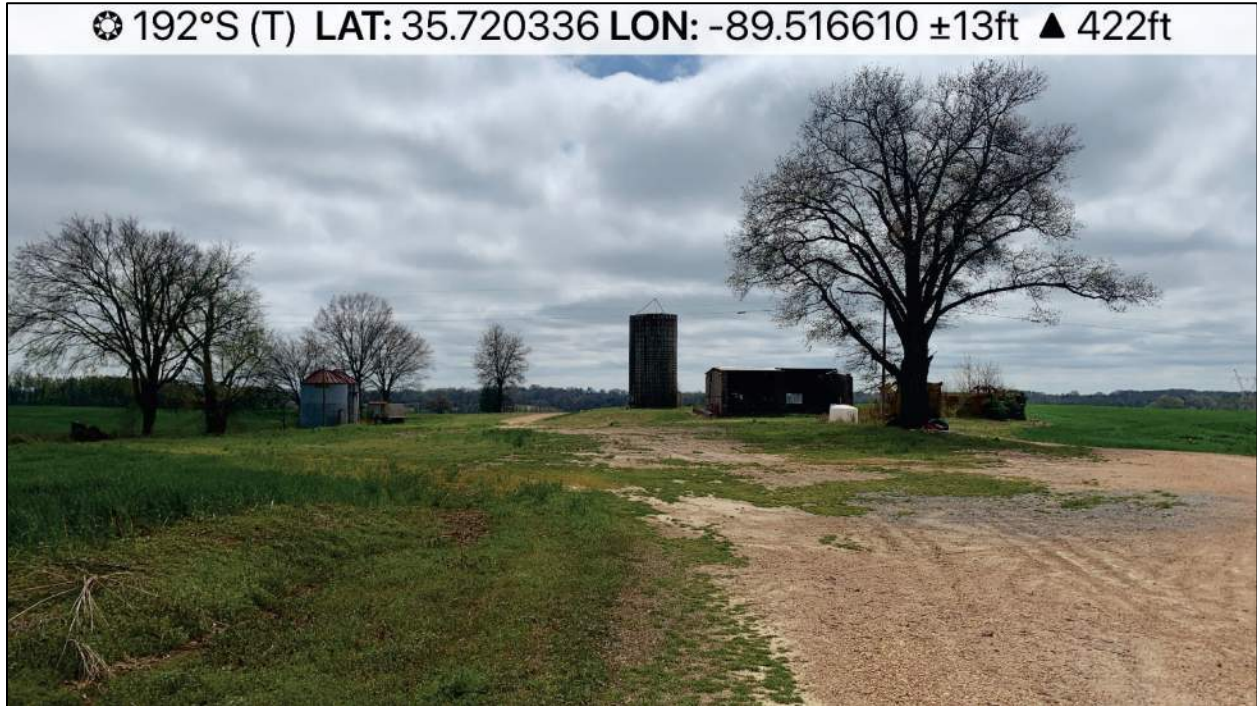
Photo 7 Facing south, general view of agricultural structures.
