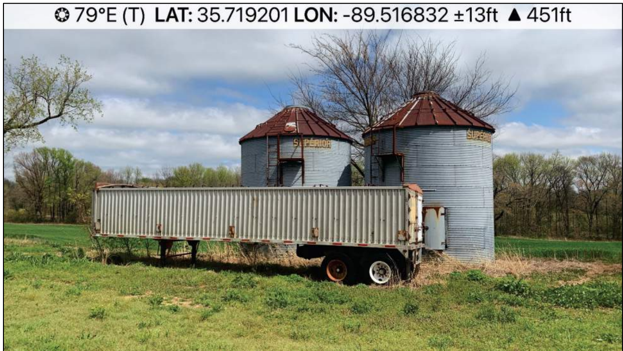
Photo 18 Facing east, semi-trailer and unused silos.
