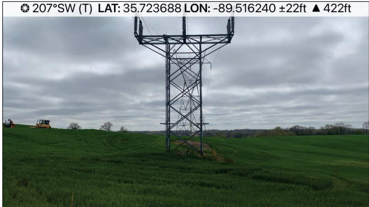
Photo 5 Facing southwest, electrical transmission towers.
