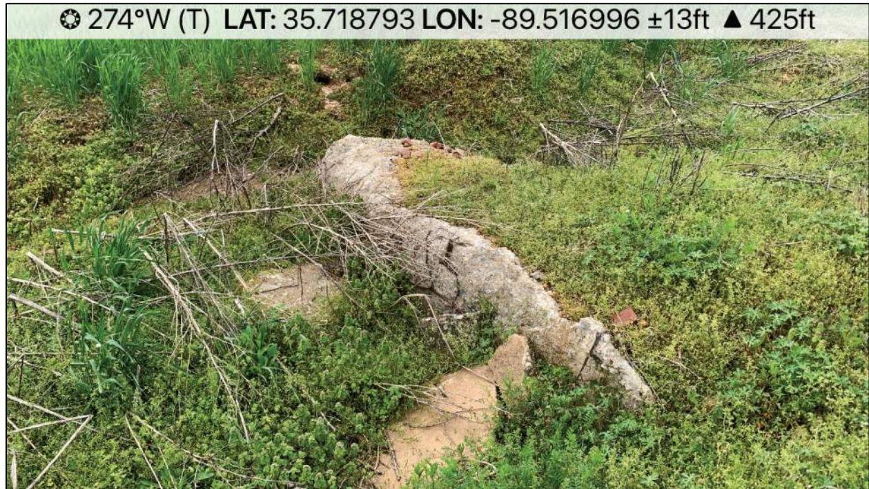
Photo 21 Facing west, concrete barriers in stream along unpaved road in southern parcel.
