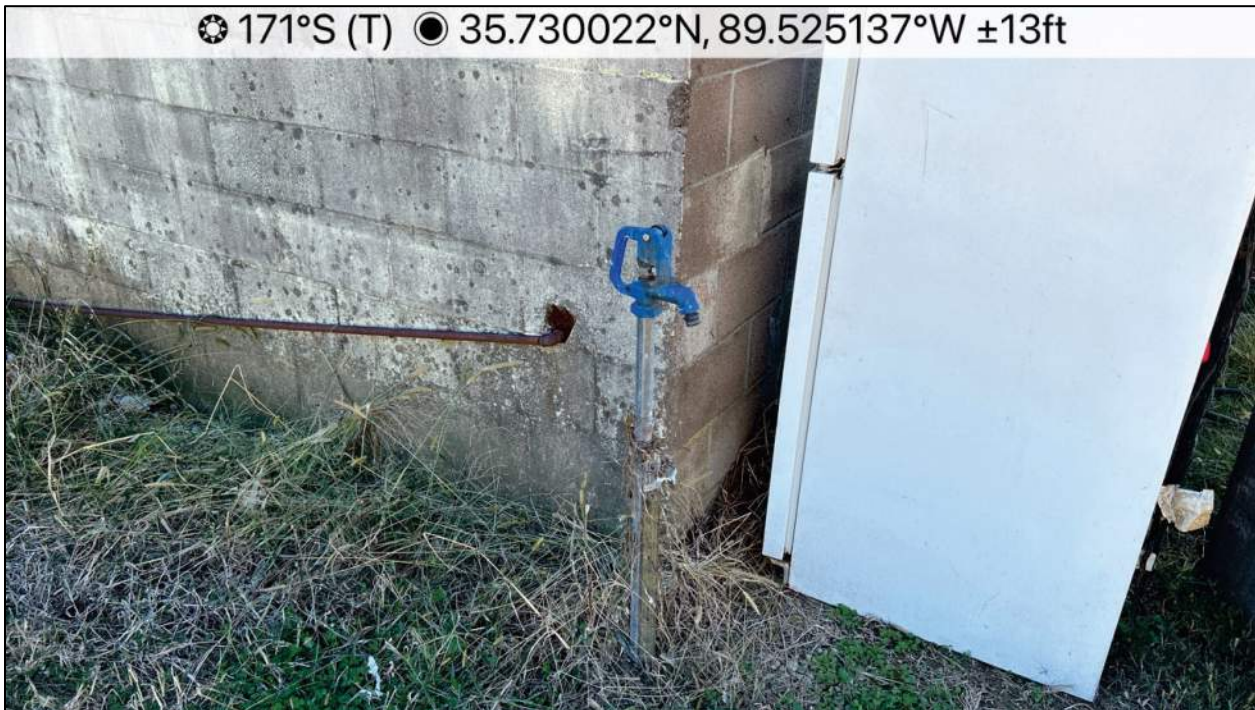
Photograph 2 – Water spigot outside abandoned structure, view to the south.
