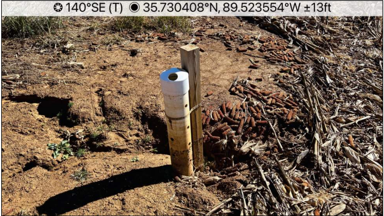
Photograph 5 – Drainage riser in the corn field, view southeast.
