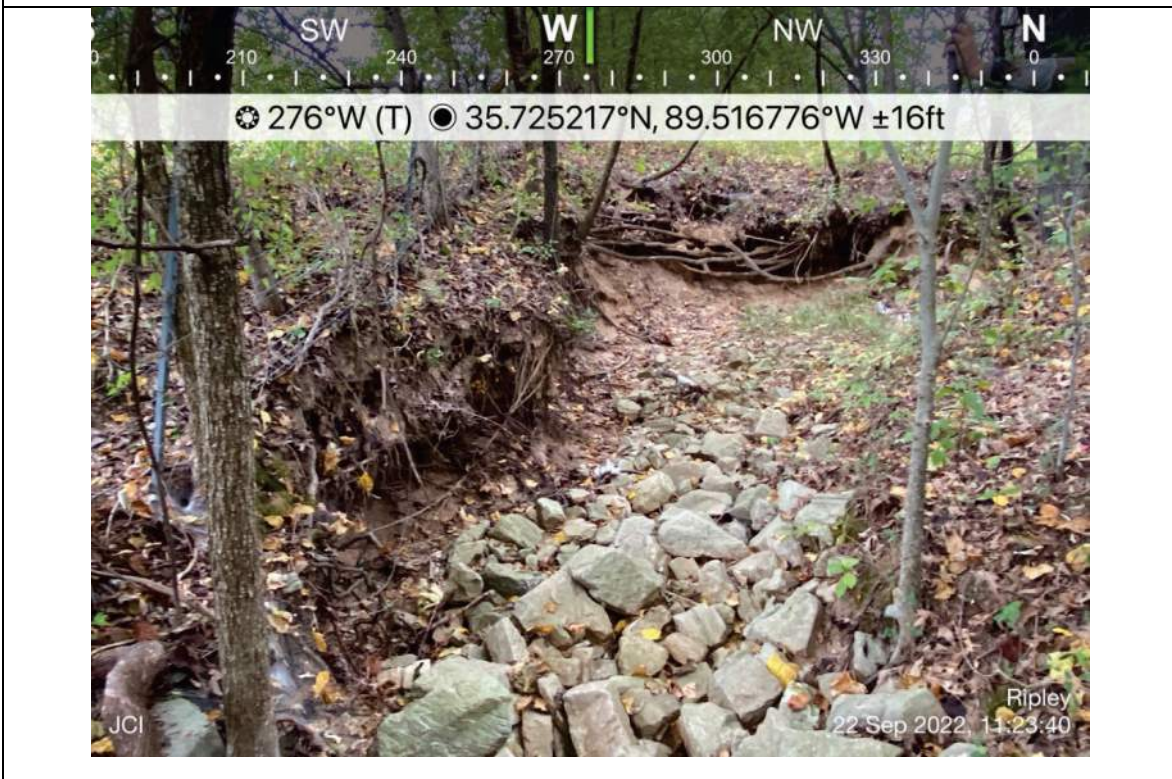
Photo 57- S016, facing west, downstream
