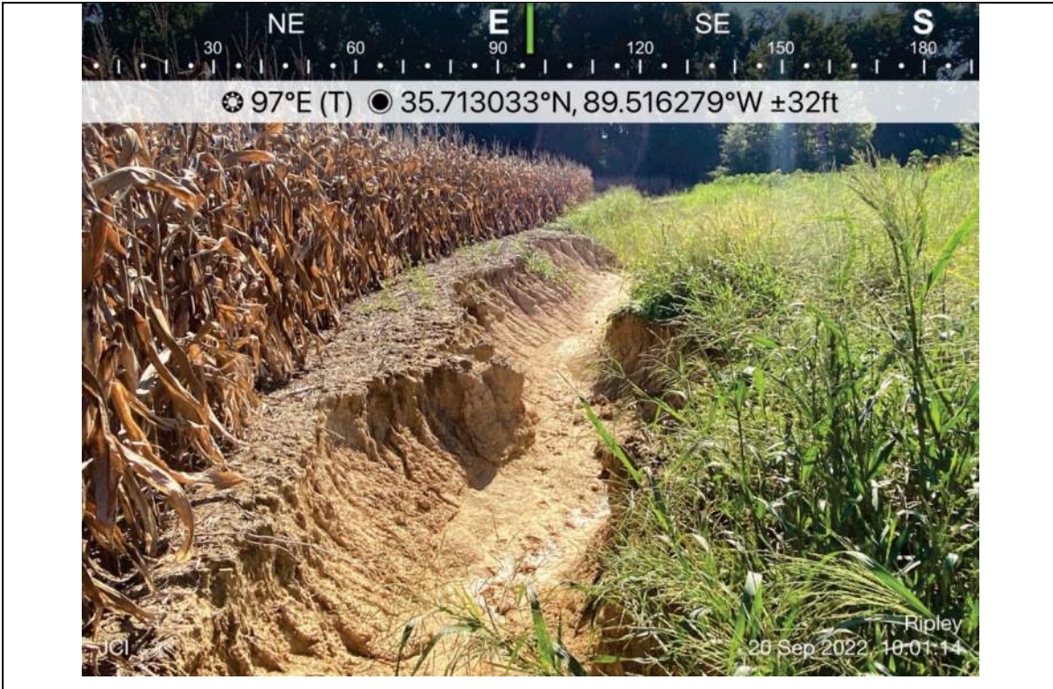
Photo 78- E009, facing east, downstream
