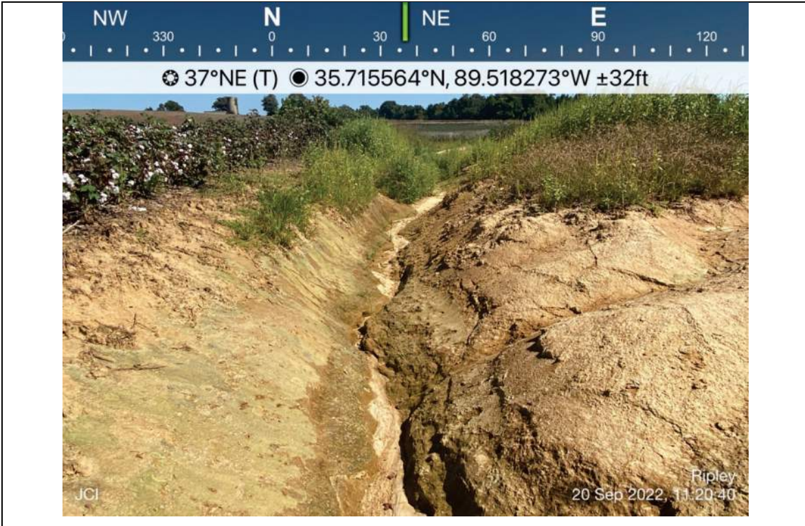
Photo 80- E011, facing northeast, downstream
