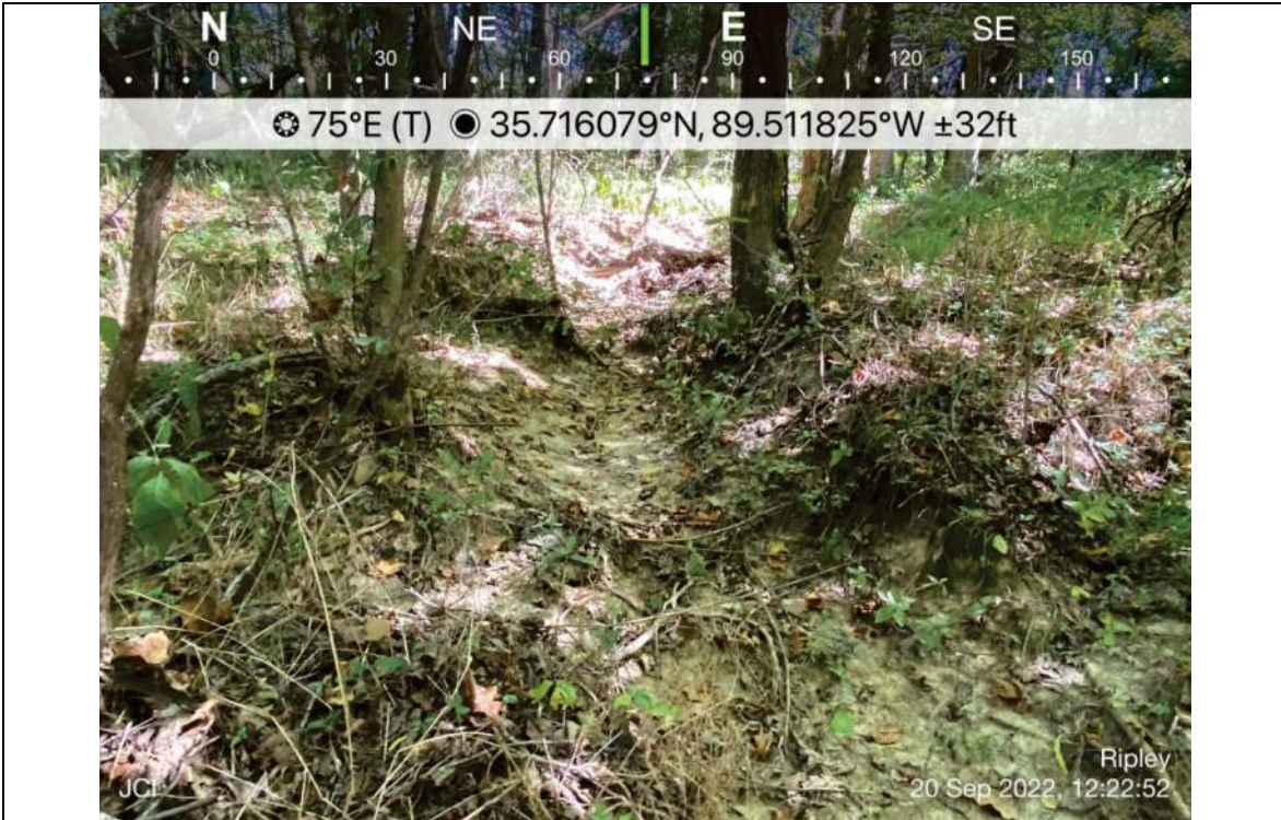
Photo 90- E016, facing east, upstream
