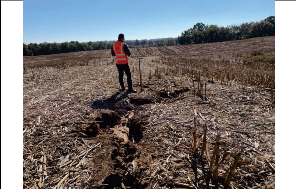
Photo 178- E061, facing southwest, downstream
