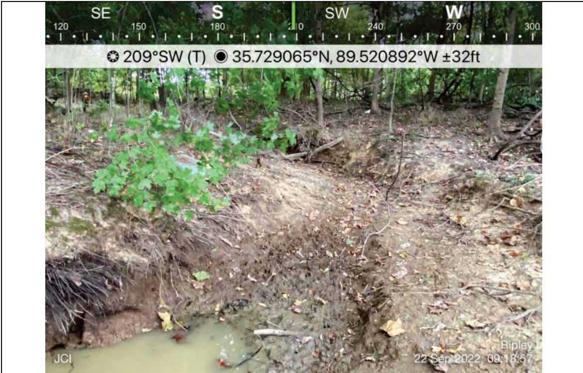
Photo 148- E046, facing southwest, downstream
