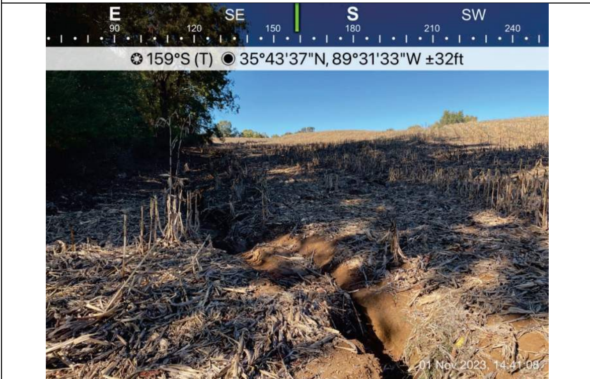
Photo 185- E065, facing south, upstream
