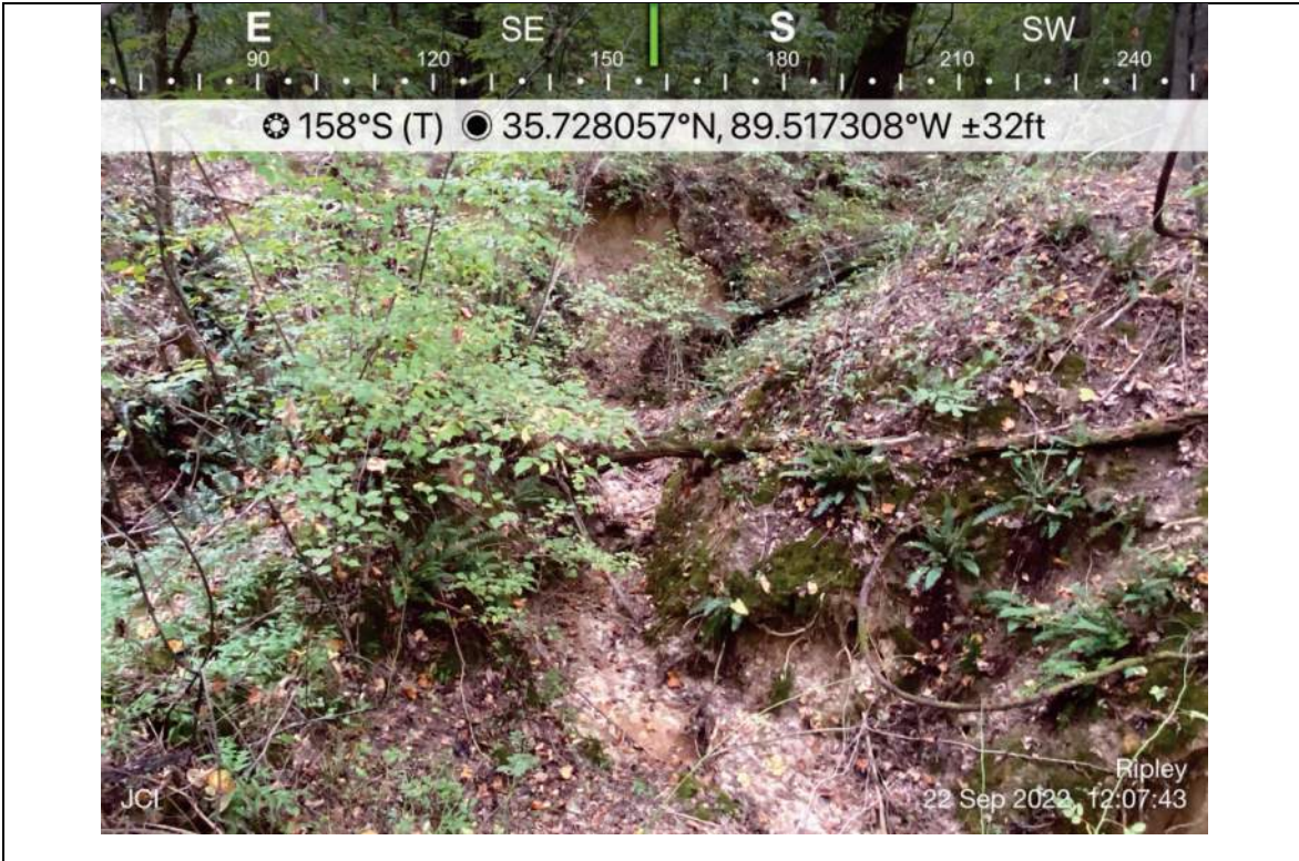
Photo 58- S017, facing south, upstream
