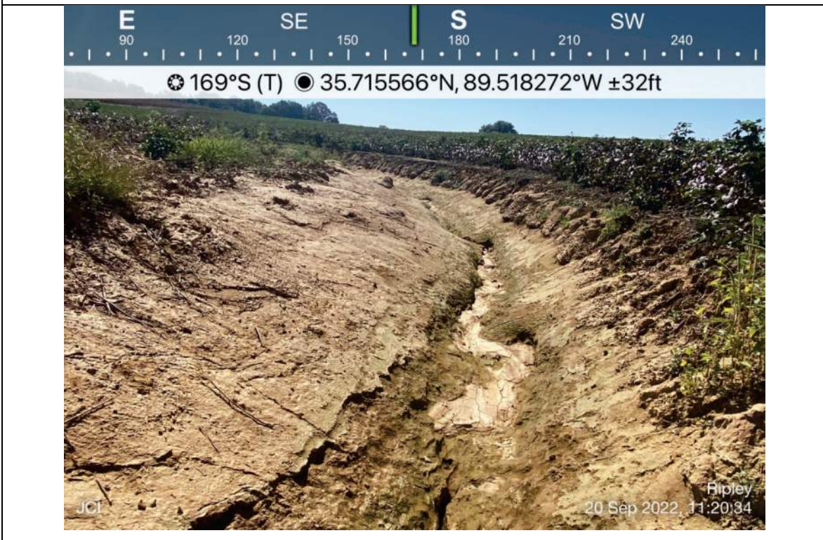
Photo 81- E011, facing south, upstream
