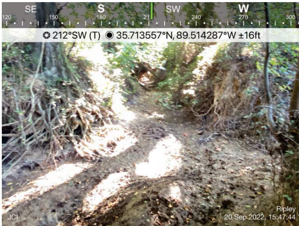
Photo 37- S006, facing southwest
