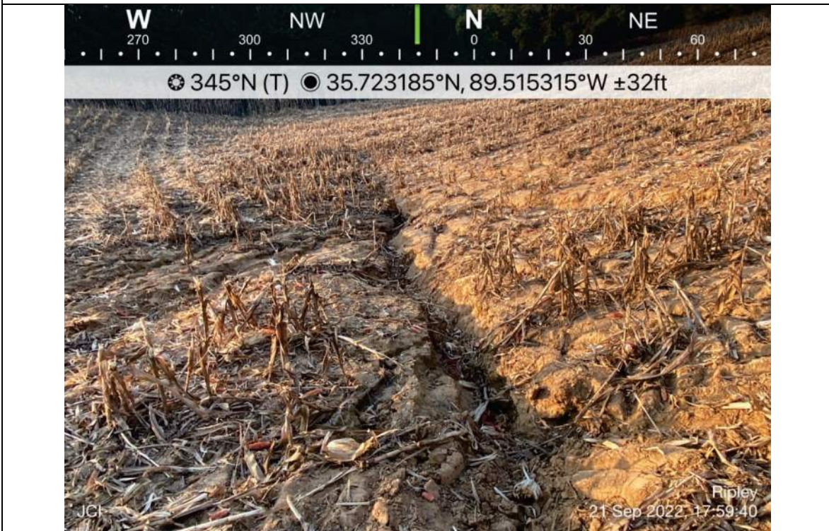
Photo 129- E036, facing north, downstream
