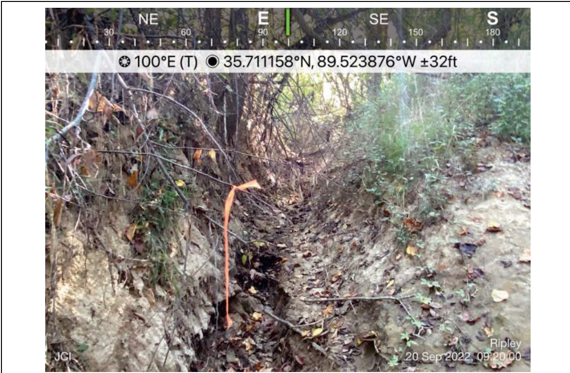
Photo 34- S005, facing east
