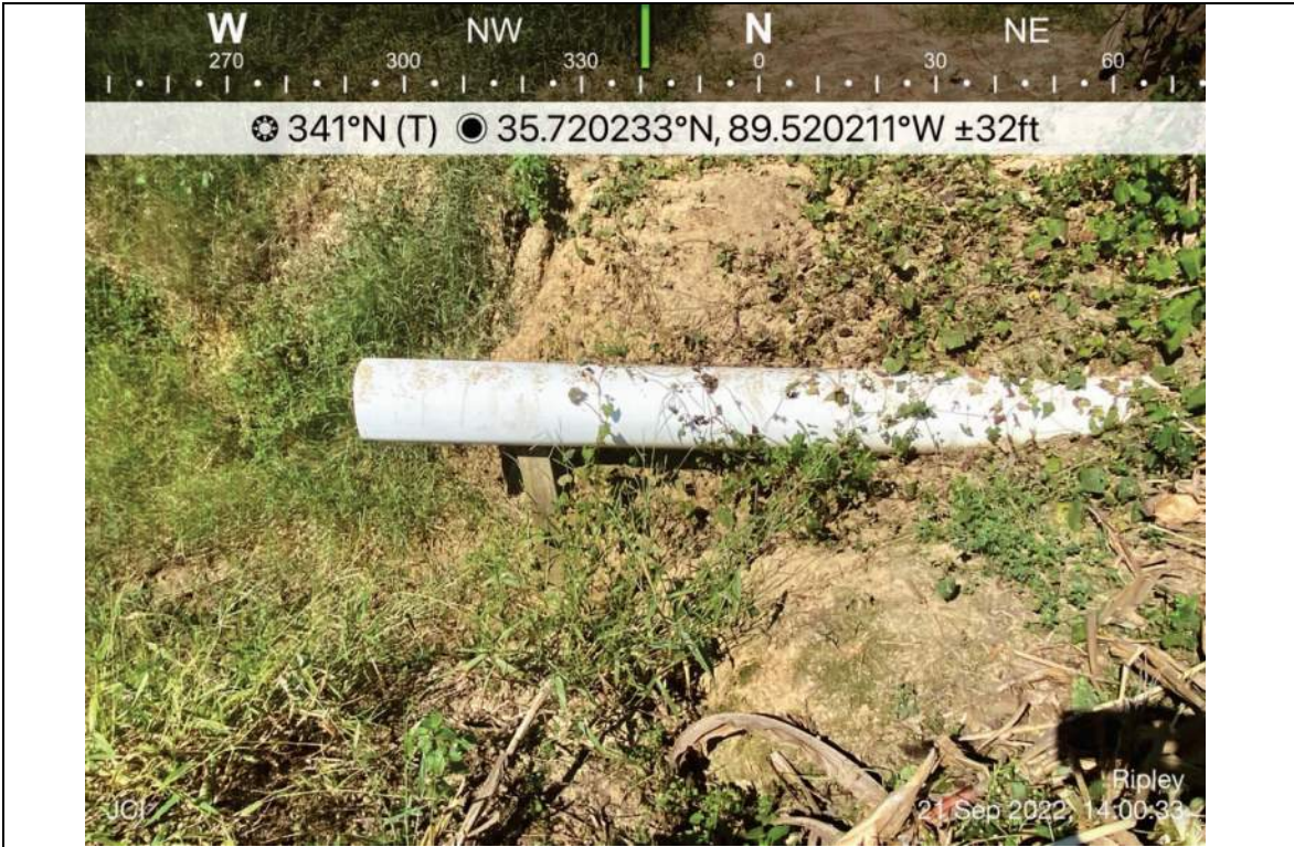
Photo 44- S010, pipe leading from Pond 1 to stream, upstream
