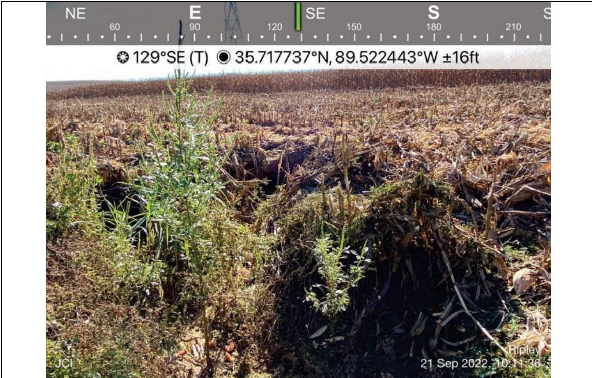
Photo 104- E023, facing southeast, upstream
