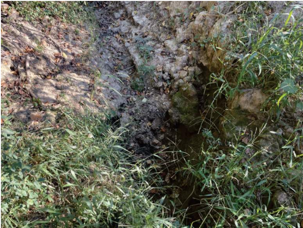
Photo 41- S008, facing downstream
