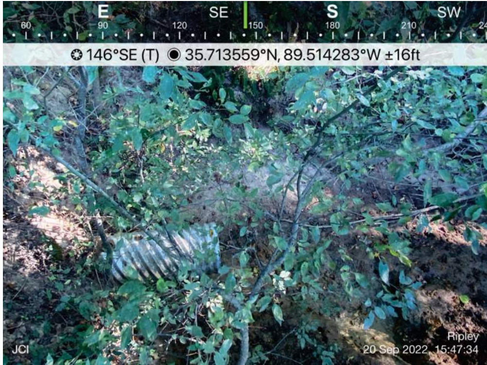
Photo 36- S006, facing southeast, culvert off property
