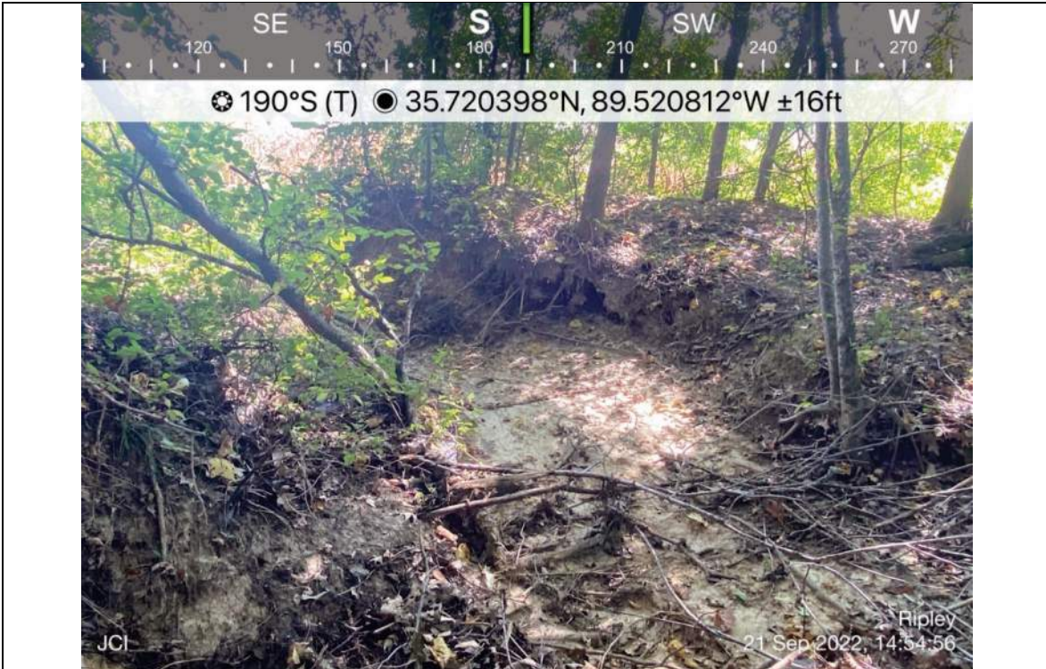
Photo 118- E030, facing south, downstream
