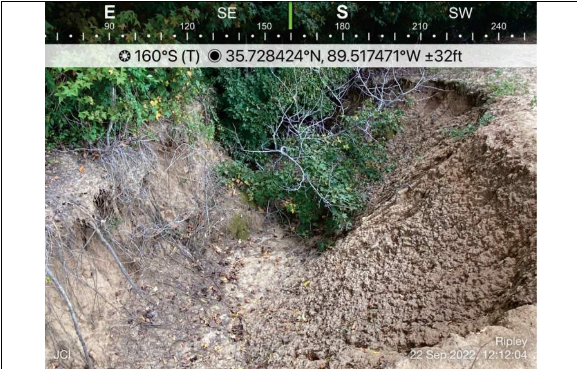
Photo 162- E053, facing south, downstream
