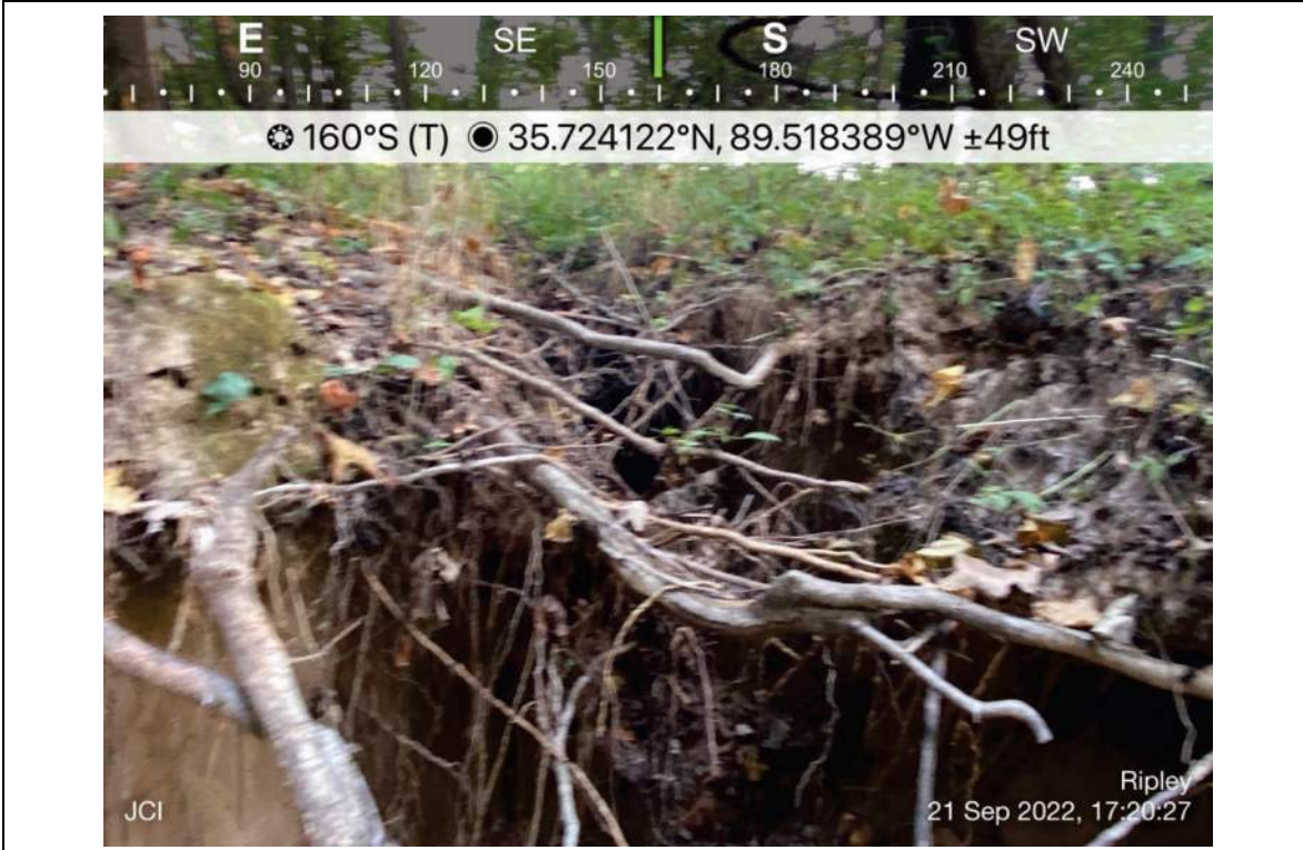
Photo 46- S011, facing southeast, upstream
