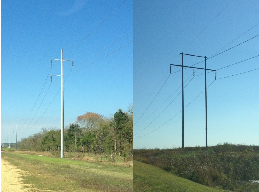
Figure 2-1 Typical Single and Double Steel-Pole Structures
