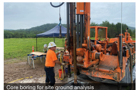
Core boring for site ground analysis
