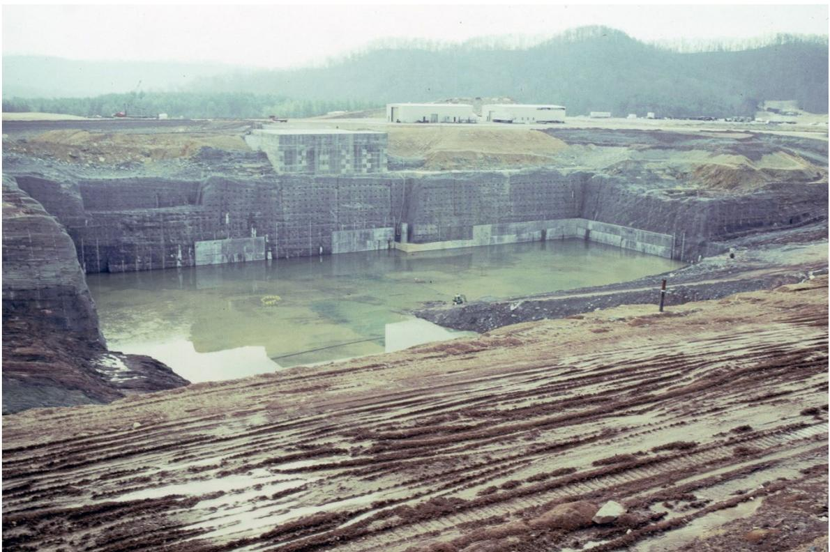
**Figure 3-22. CRBRP Grading and Excavation**
