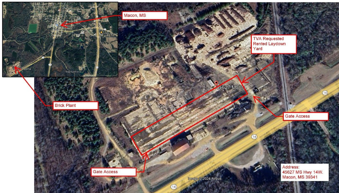
Figure 2-1. Macon, Mississippi Brickyard Laydown Area
