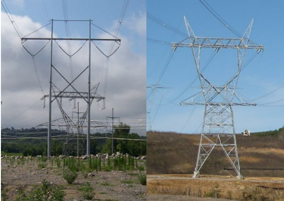
Figure 2-2. Examples of 500-kV Transmission Structures
