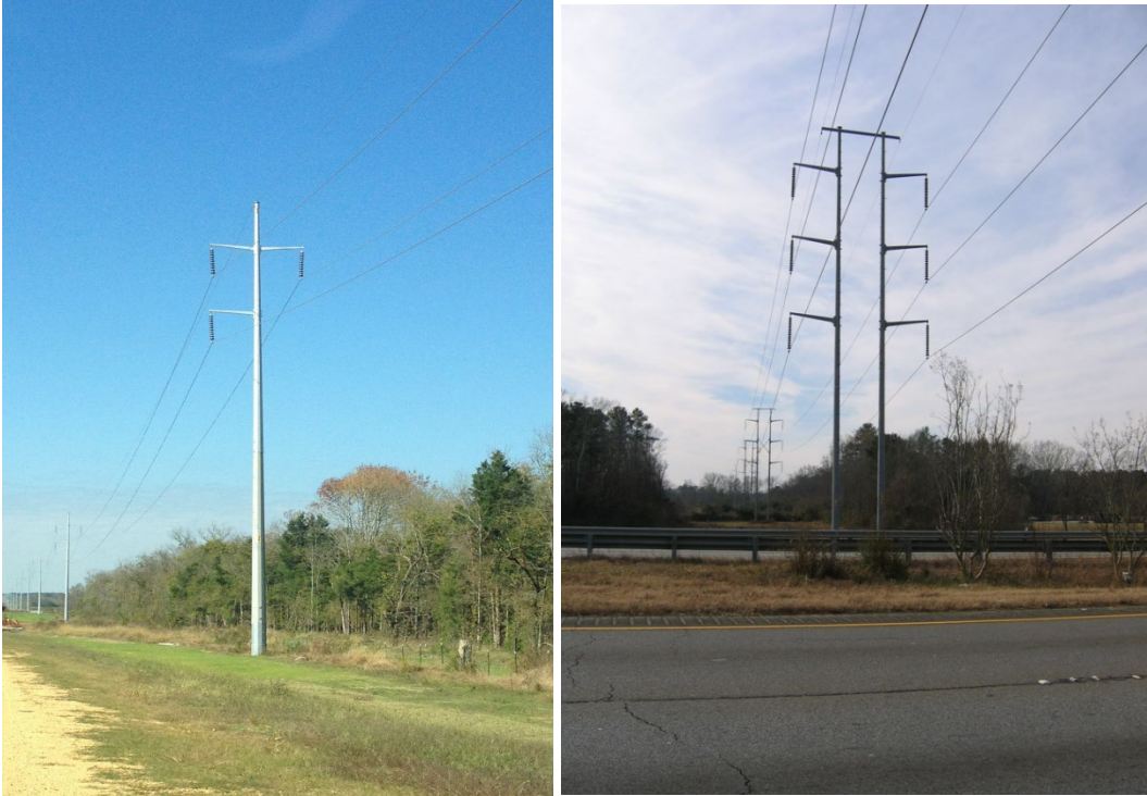
Figure 2-4. Typical Single and Double Steel-Pole Structures
