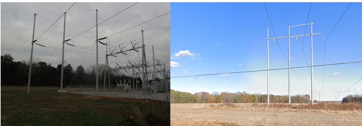
Figure 2-5. Typical Triple Steel-Pole Structures
