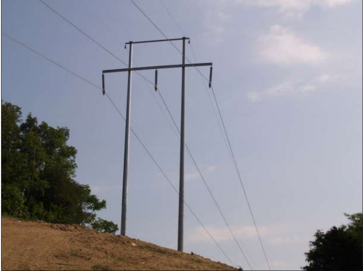
Figure 2. Typical example of the type of transmission line structure that would be installed.
