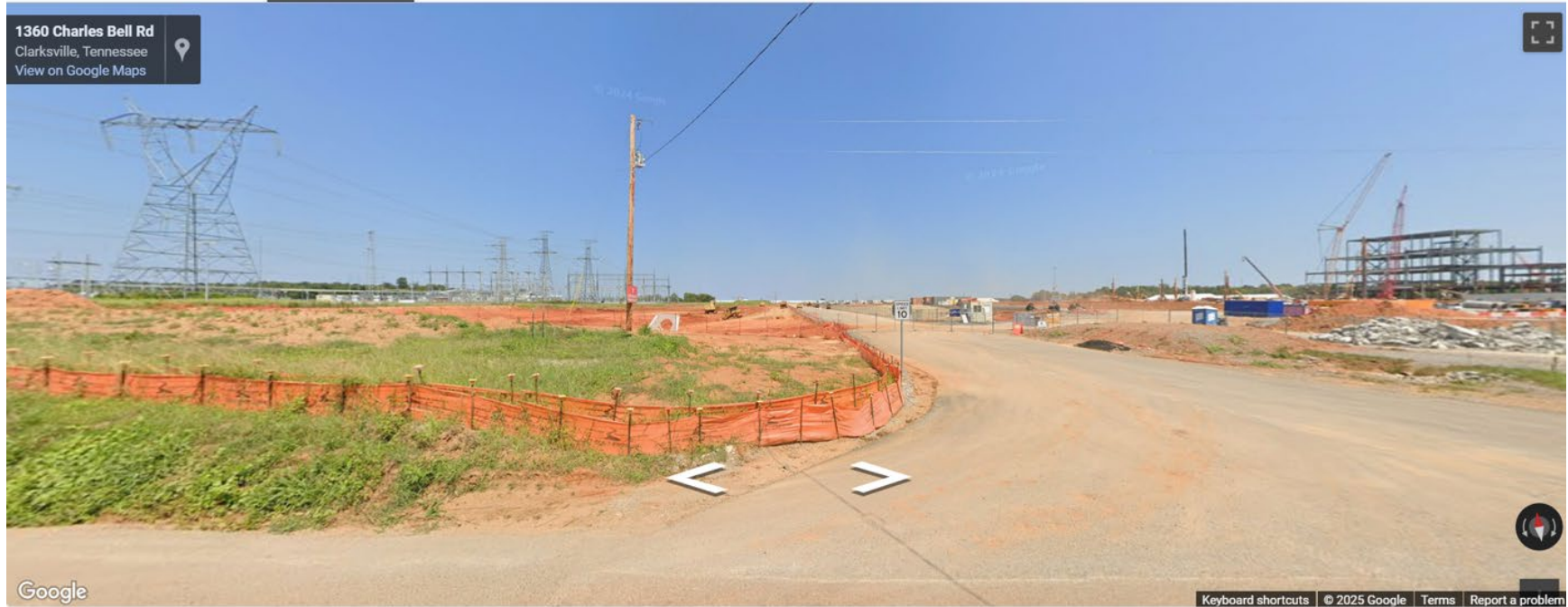
View North from Parcel 2 on Charles Bell Road, Montgomery County, Tennessee
