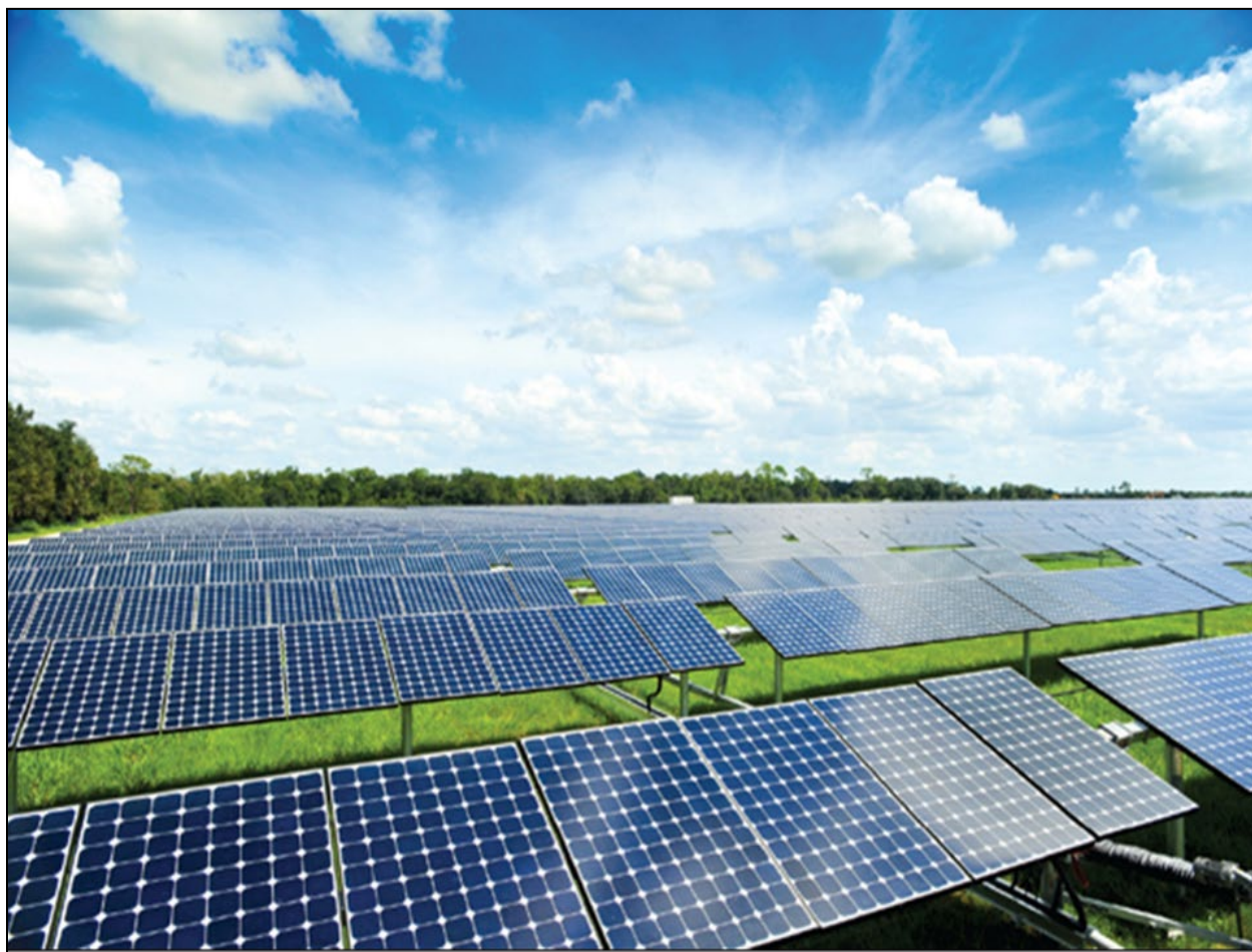
Photo 3.5-5. Single-axis, tracking photovoltaic system with panels close to maximum tilt
