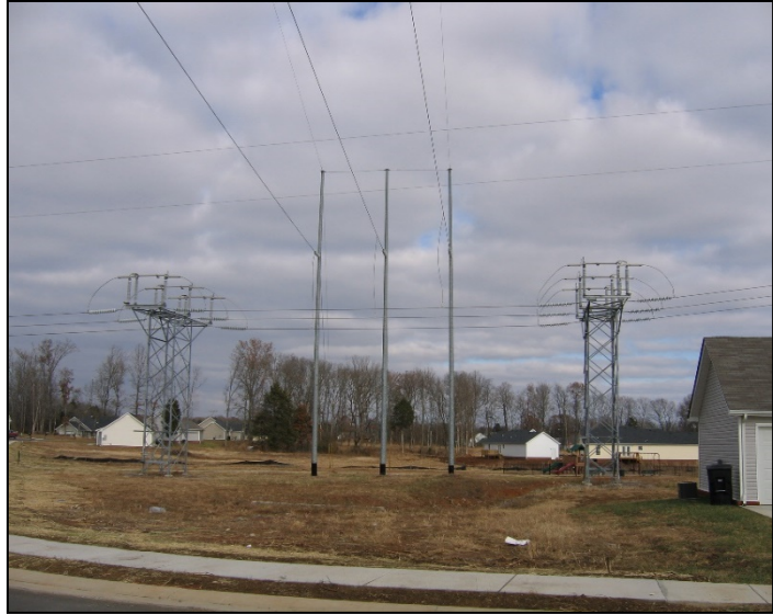
Photo 2-3. Example of switch structures and associated 3-pole transmission structure at a transmission line tap point
