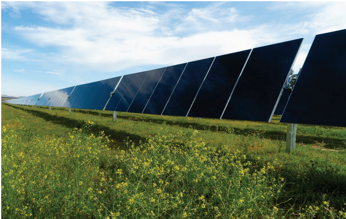
Figure 3-34. Single-axis, tracking photovoltaic system with panels near maximum tilt as viewed from the east or west
