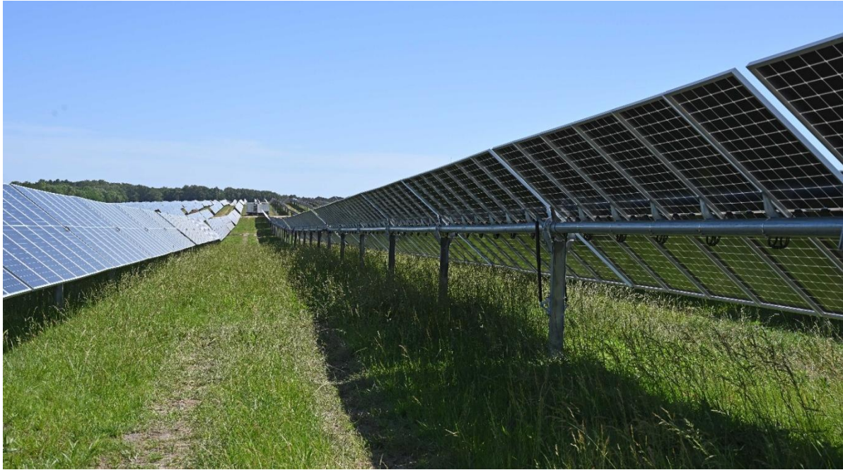
Figure 3-23. Typical arrangement of PV arrays.
