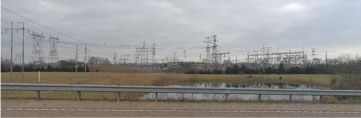
Figure 3-16. Existing Conditions View South toward West Point Substation from Yokohama Boulevard
