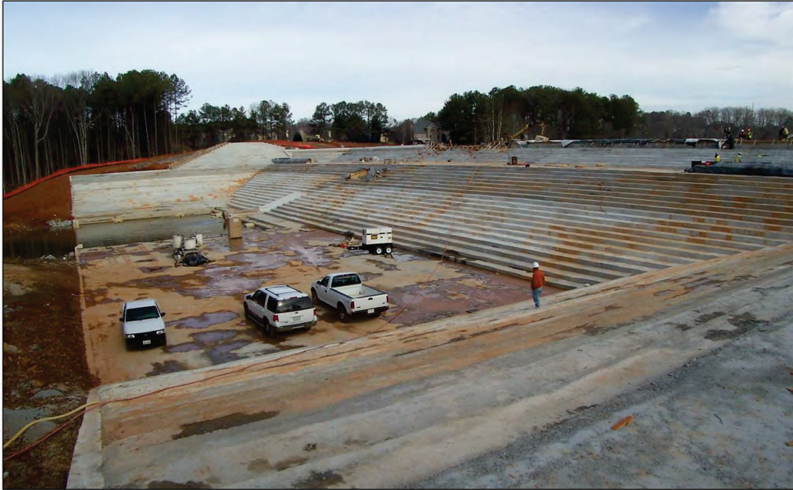
Figure 2.1-12. Typical completed RCC structure.
