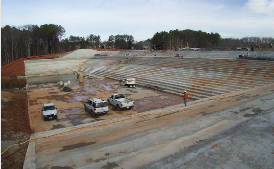
Figure 2.1-12. Typical completed RCC structure.
