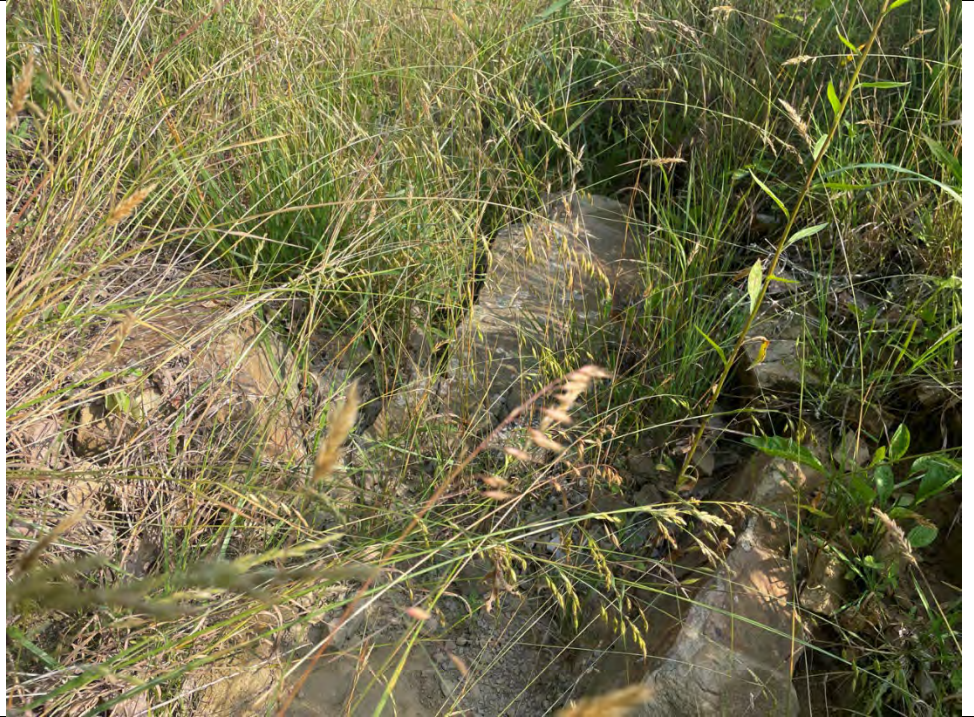
157. E004, facing upstream and northwest
