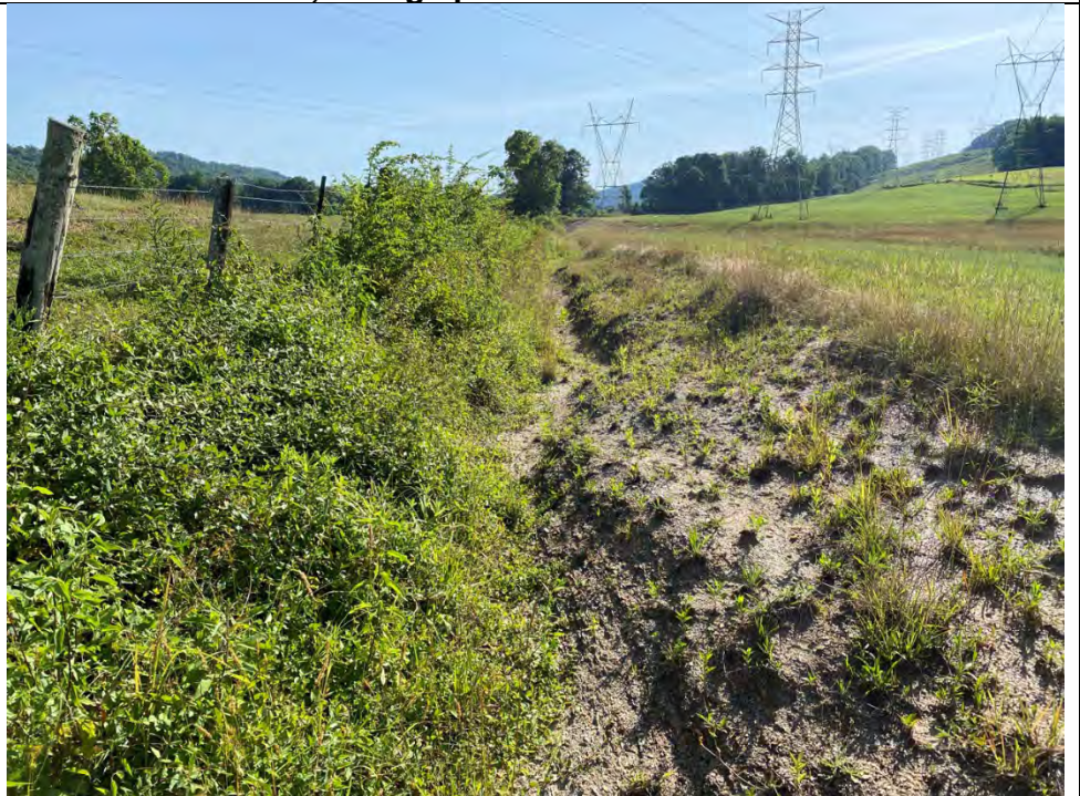
162. E007, facing upstream and northwest
