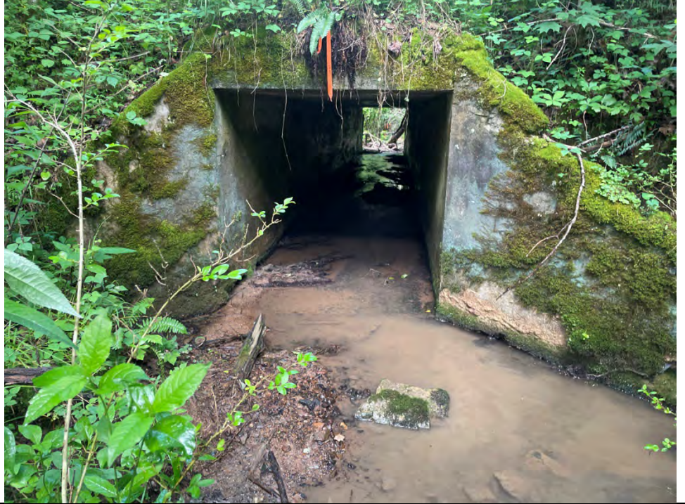
112. S033 (Perennial), facing downstream and east
