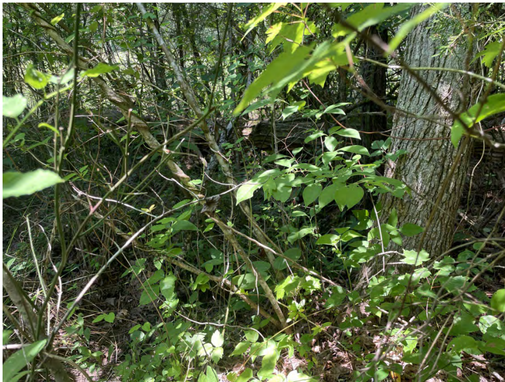
Photo 252. E128, Erosional Gully, facing downstream and northwest.
