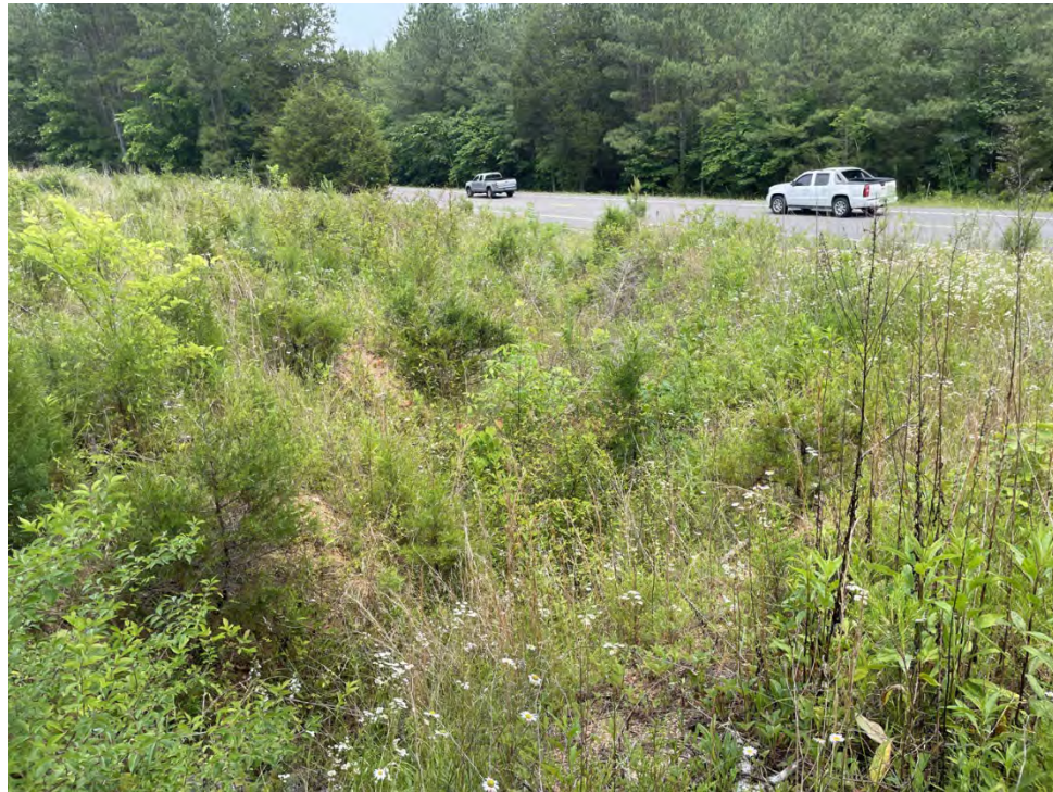
Photo 254. E129, Erosional Gully, facing downstream and east.
