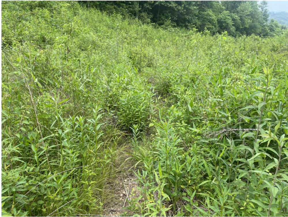
Photo 247. E126, Erosional Gully, facing downstream and north.
