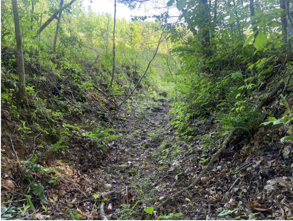
Photo 235. E117, Erosional Gully, facing upstream and northwest.
