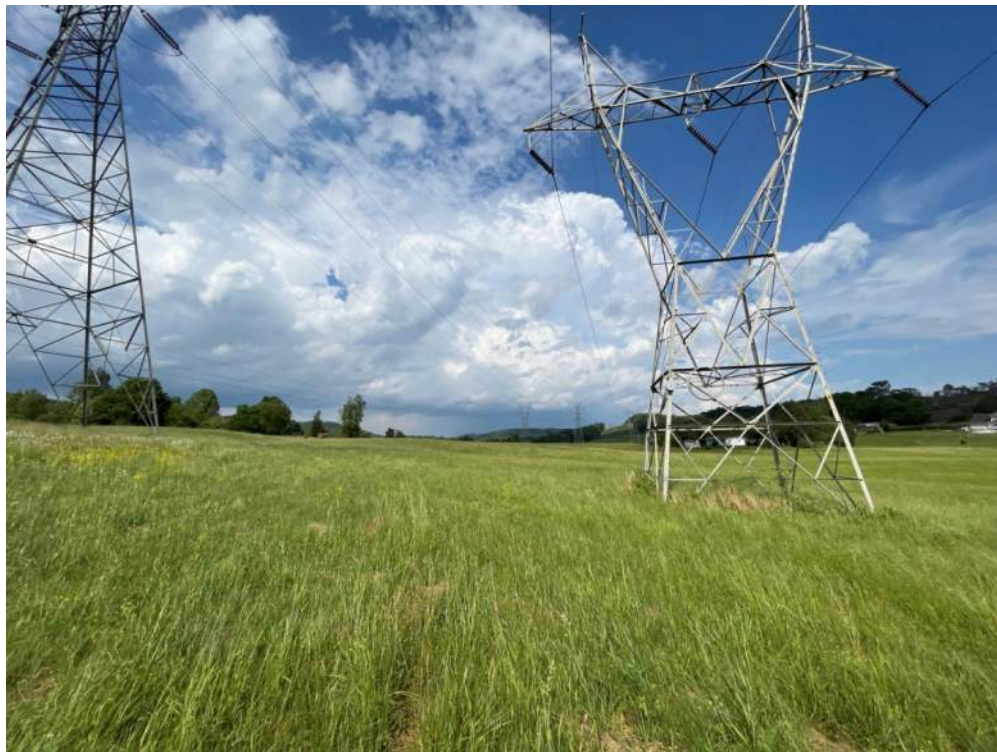
Photo 6- Representative of maintained lawn within Project site, facing east.
