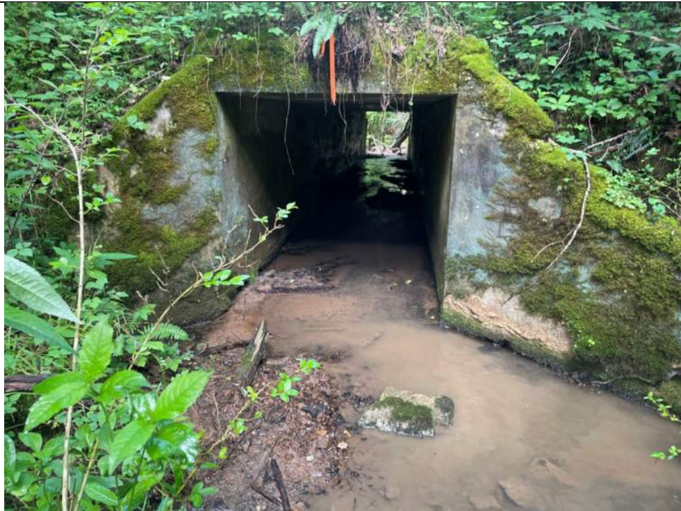
Photograph 36- Forest Stand 20 box culvert and water resource within stand, facing west.
