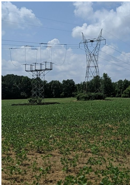
Photo 2.2-1. Existing steel tower structure and switch
