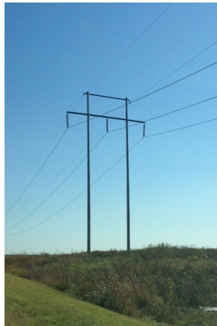
Photo 2.2-2. Proposed steel pole structure
