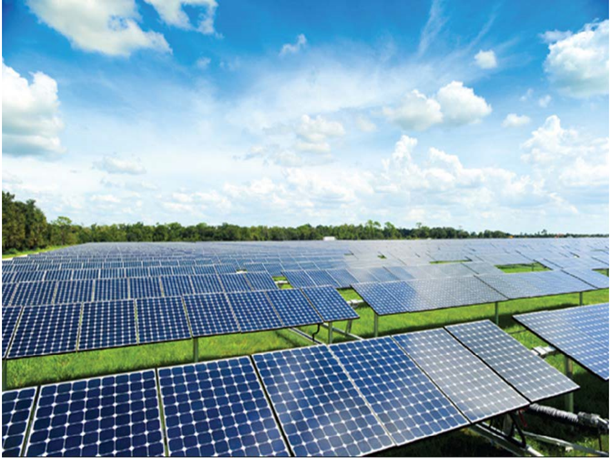
Photo 3.5-6. Single-axis, tracking photovoltaic system with panels showing some tilt as viewed from the east or west
