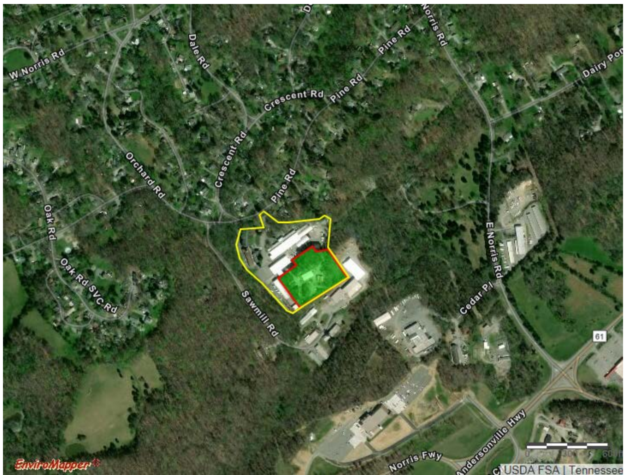
Figure 1. Engineering Lab Property (approximate property boundary in yellow) with Phase 1 construction and soil removal area highlighted in green (with red outline)
