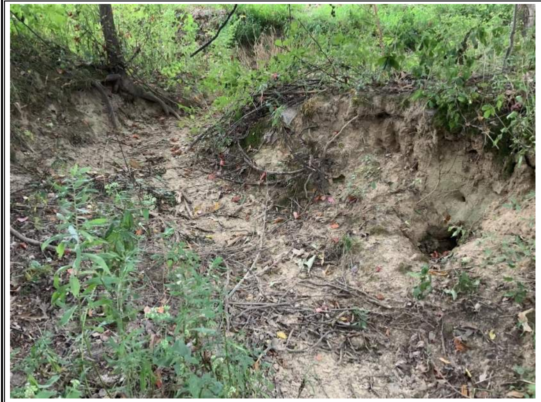
Photo: 50 By: F. Amatucci Date: September 22, 2022 Feature: ES-8 Lat: 36.443848 Long: -88.304328
