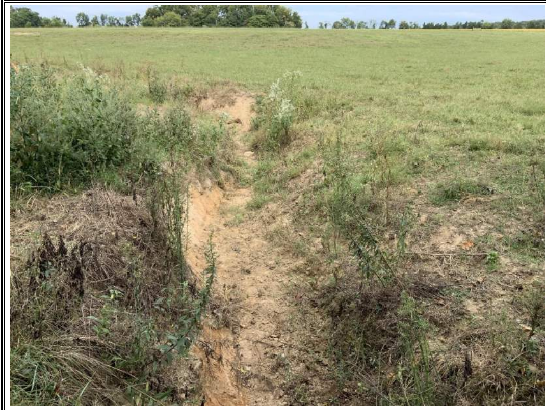
Photo: 52 By: F. Amatucci Date: September 22, 2022 Feature: ES-10 Lat: 36.441588 Long: -88.297518
