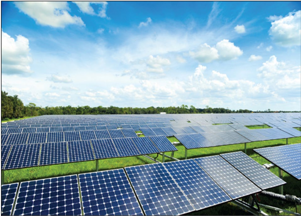
Photo 3.5-6. Single-axis, tracking photovoltaic system with panels close to maximum tilt
