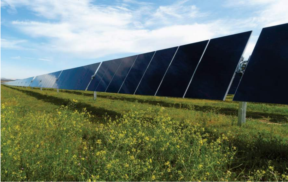
Figure 3-15. Single-axis, tracking PV system with panels near maximum tilt as viewed from the east or west
