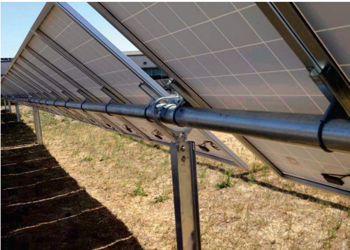
Figure 3-16. The backside of the solar panels in early morning or late afternoon configuration
