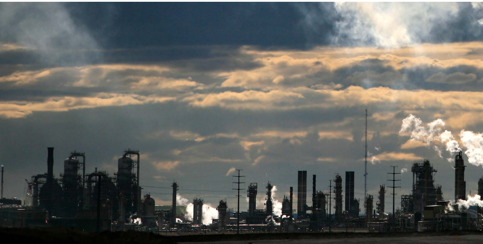
Syncrude upgrader plant north of Fort McMurray, Alberta, Canada
