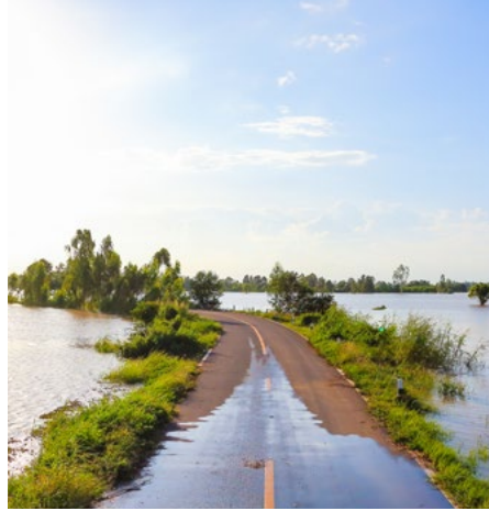
Coastal road networks and the communities they support are increasingly at risk of impacts from sea level rise and intensifying coastal flood events.
