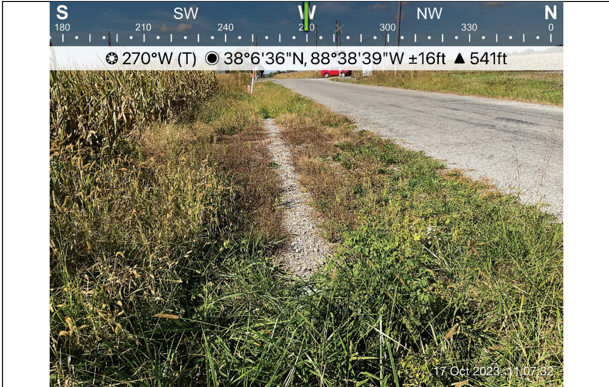
Photo 9- Culvert parallel to E005.
