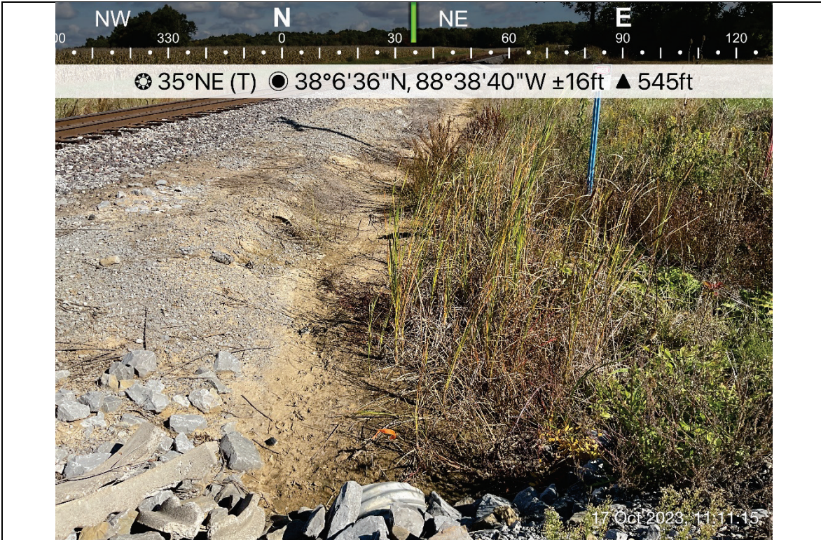
Photo 15- Culvert underneath railroad tracks at intersection with CR 350 East.
