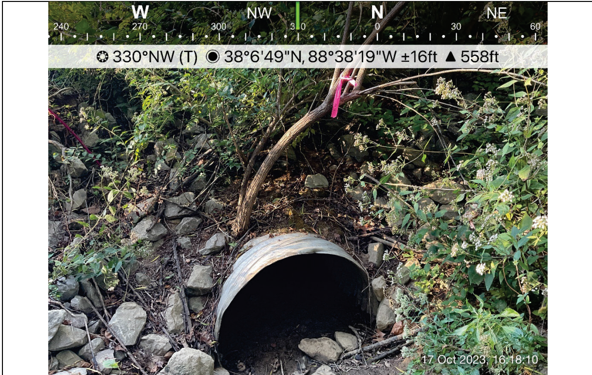
Photo 3- Culvert underneath railroad track, where E010 flows into S002.
