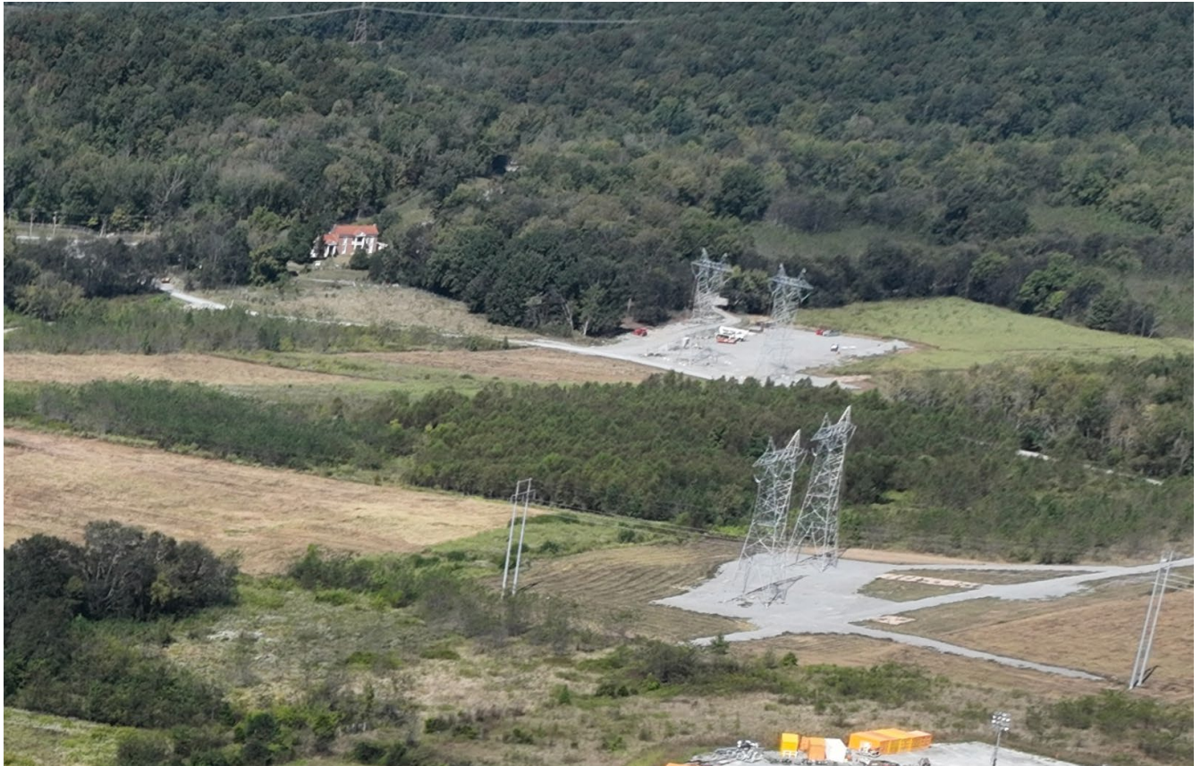
Figure 8 - Crop of above image showing SW-745 in relation to existing and planned infrastructure.
