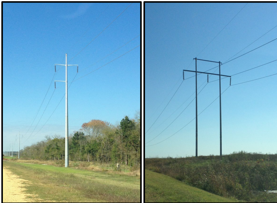
Figure 2-2. Typical 161-kV Single and Double Steel-Pole Structures
