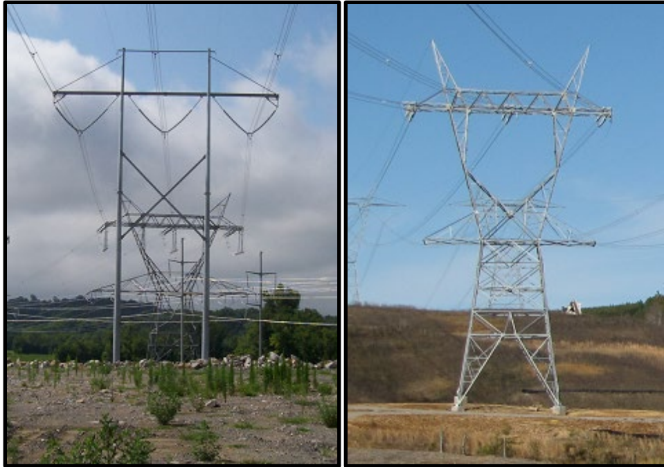
Figure 2-1. Typical 500-kV H-Frame and Laced Steel-Pole Structures
