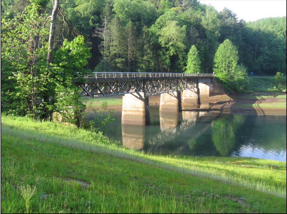
Figure 2. The existing Wilbur Reservoir Bridge, carrying Wilbur Dam Road over Wilbur Reservoir
