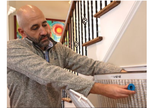
Brad Wagner, manager of program operations at TVA EnergyRight, installs a whistle that emits a sound when a furnace filter needs to be changed.
