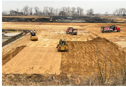
Making significant progress on the East Ash Disposal Area
