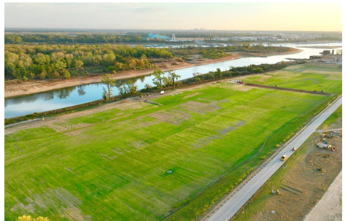
Coal ash removal at West Ash Disposal Area is complete.
