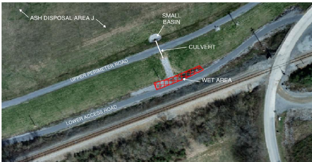
Figure 1. Aerial View of 2019 Wet Area
