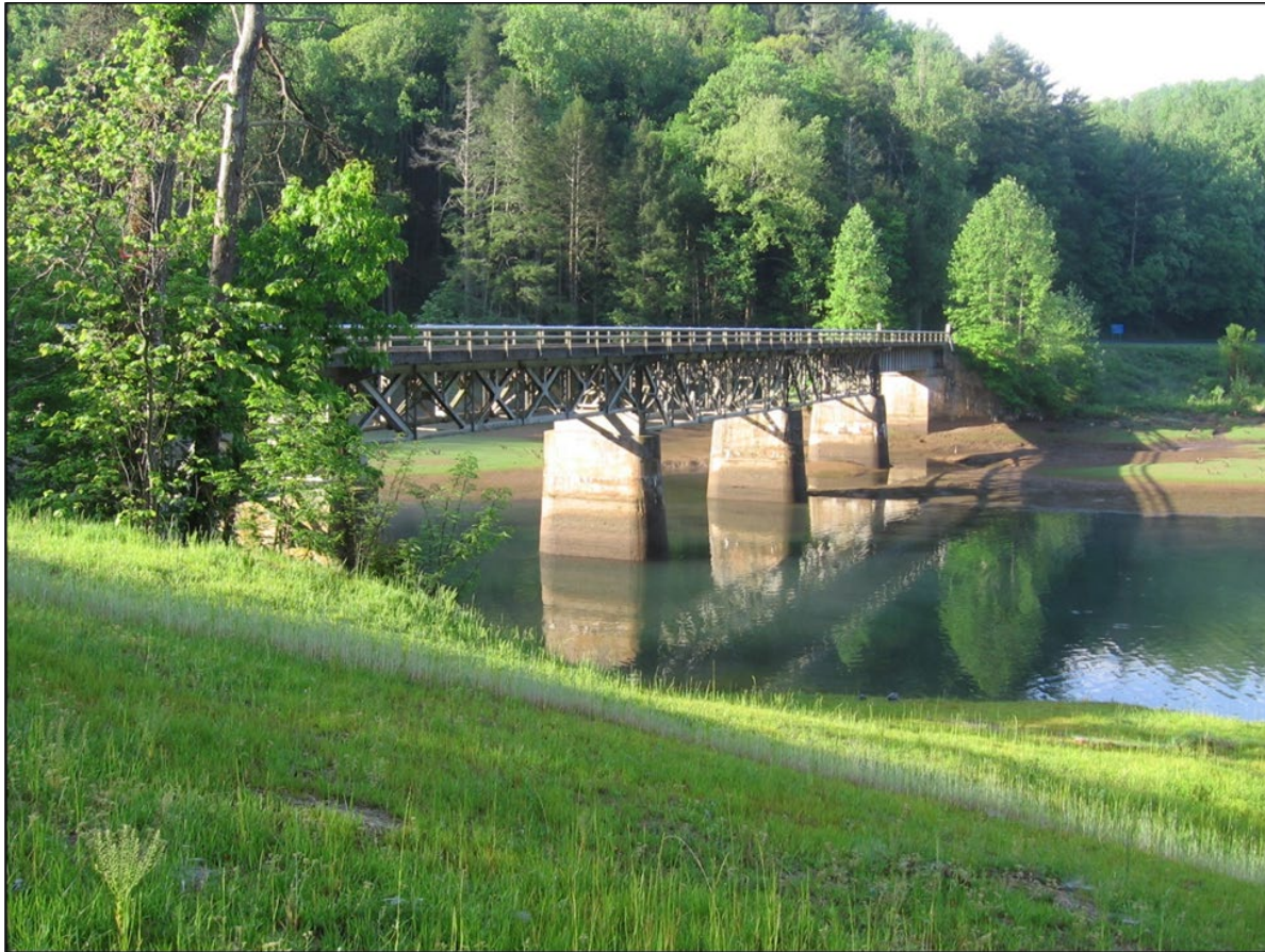
Figure 2. The existing Wilbur Reservoir Bridge, carrying Wilbur Dam Road over Wilbur Reservoir
