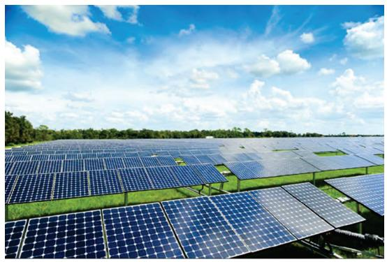
Photo 3-15. Single-axis, Tracking PV System with Panels Showing Some Tilt as Viewed from the East or West
