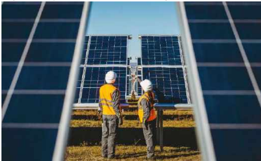
Figure 3-10: Representative Photo of Single-Axis Tracking PV System in the Morning, Facing East
