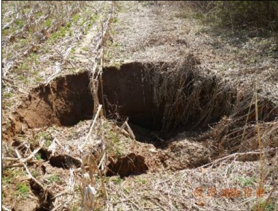
Figure 3.8 Representative Photograph of Open-Throat Sinkhole Feature Encountered During Karst Survey
