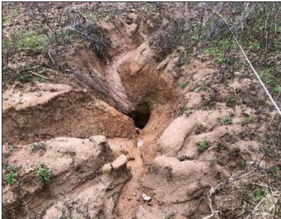
Figure 3.9 Representative Photograph of Open-Throat Sinkhole Feature Encountered During Karst Survey
