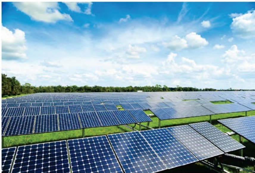
Figure 3-12. Single-axis, tracking photovoltaic system with panels showing some tilt as viewed from the east or west.
