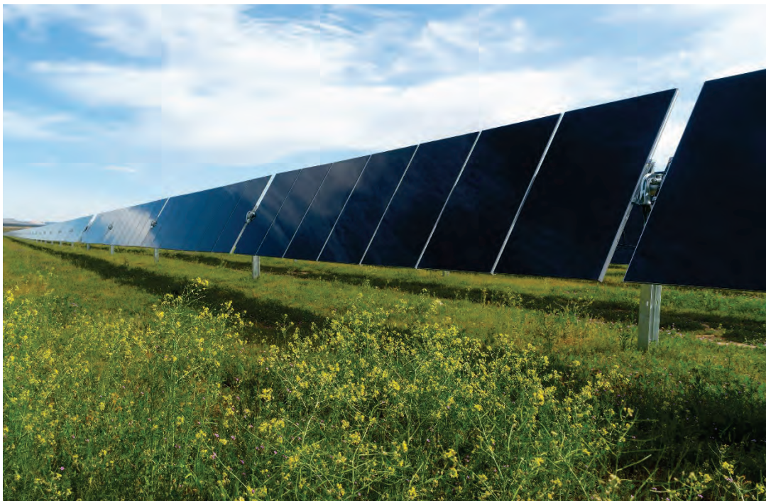
Photo 3-5. Single-axis, tracking photovoltaic system with panels near maximum tilt as viewed from the east or west
