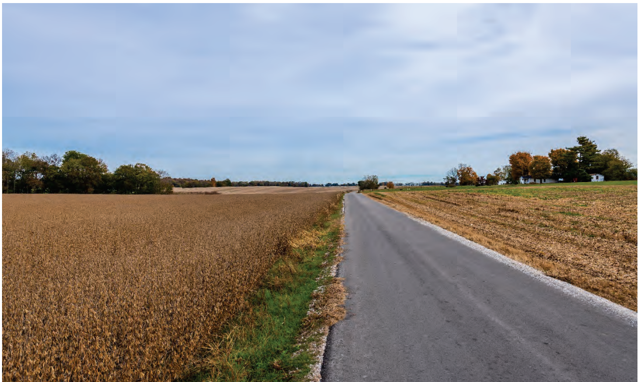
Photo 3-4. View to Project site looking east along AP Miller Road, about 100 yards east of Watermelon Road
