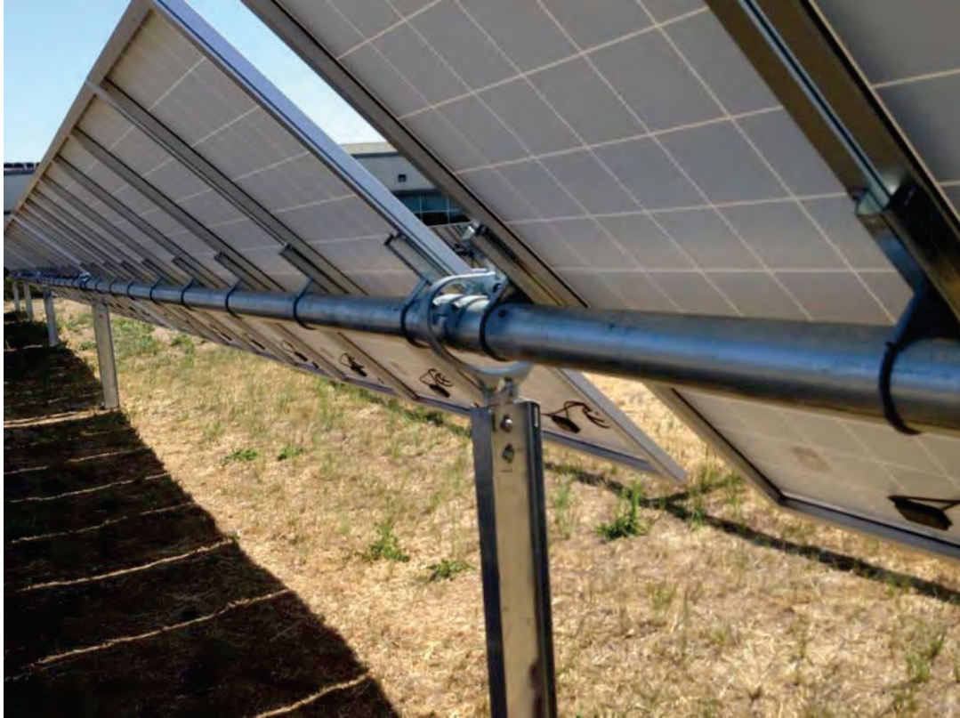
Photo 3-6. The backside of the solar panels in early morning or late afternoon configuration
