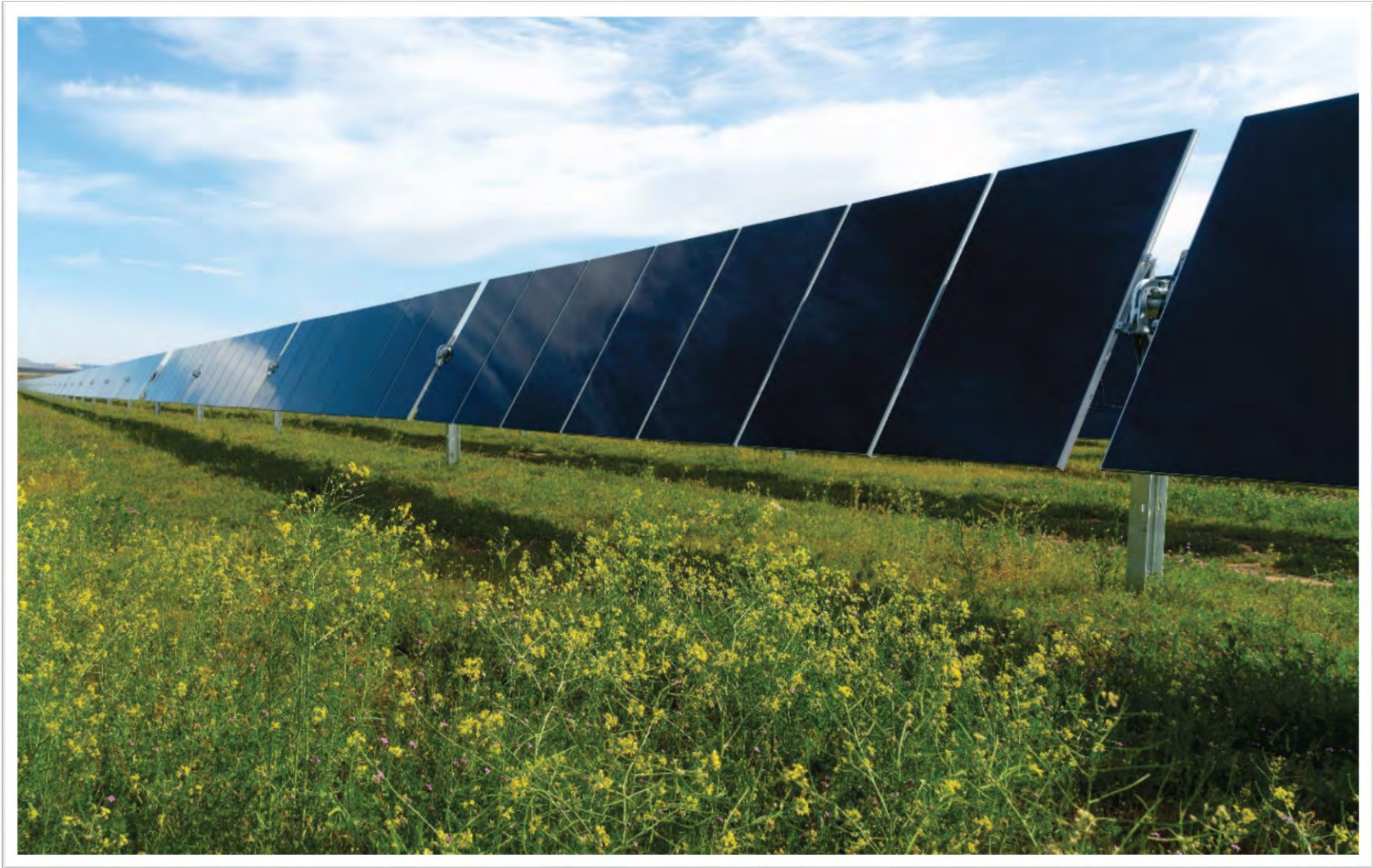
Figure 1: Example of a single-axis, tracking photovoltaic system with panels near maximum tilt as viewed from the east or west.
