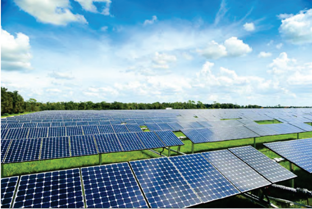
Photo 3-13. Single-axis, tracking photovoltaic system with panels showing some tilt as viewed from the east or west
