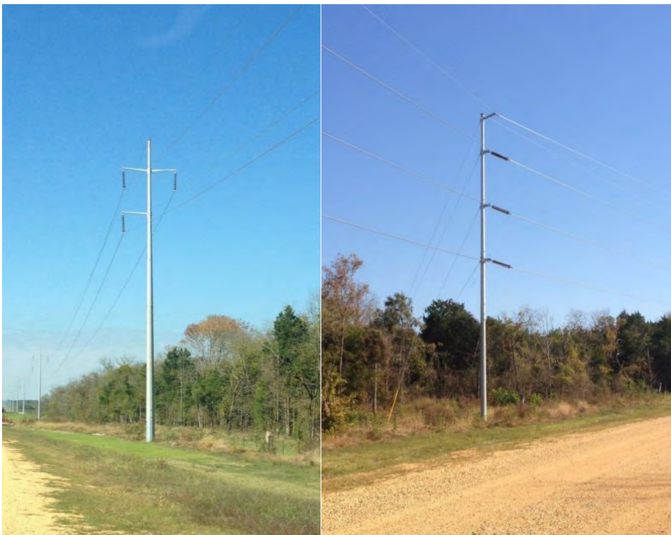
Figure 2-1. Typical Single-Circuit Steel-Pole Transmission Line Structure
