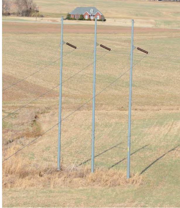
Figure 2-2. Typical Single-Circuit Steel Three-Pole Transmission Line Structure
